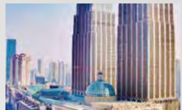
Toppan (Shanghai) Management Co., Ltd. (Shanghai, China)
